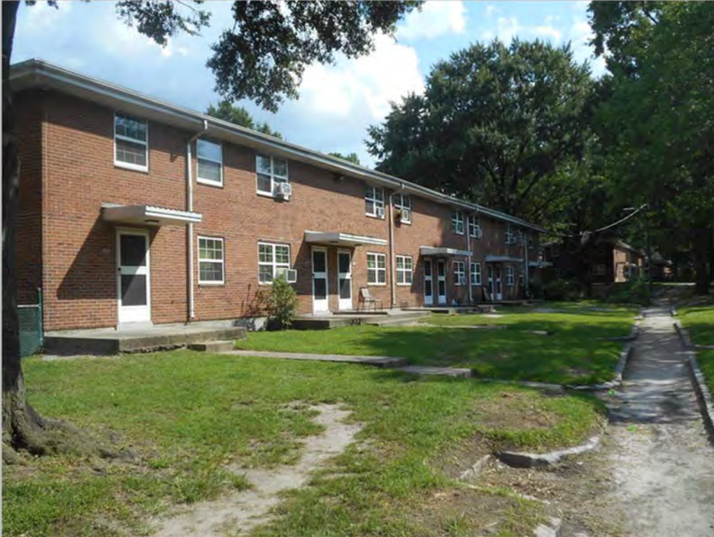
Typical building exterior front elevation
