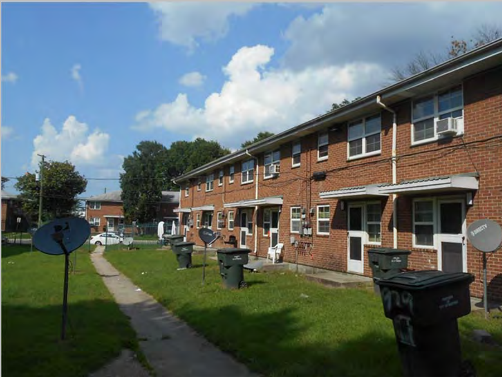
Typical building exterior rear elevation
