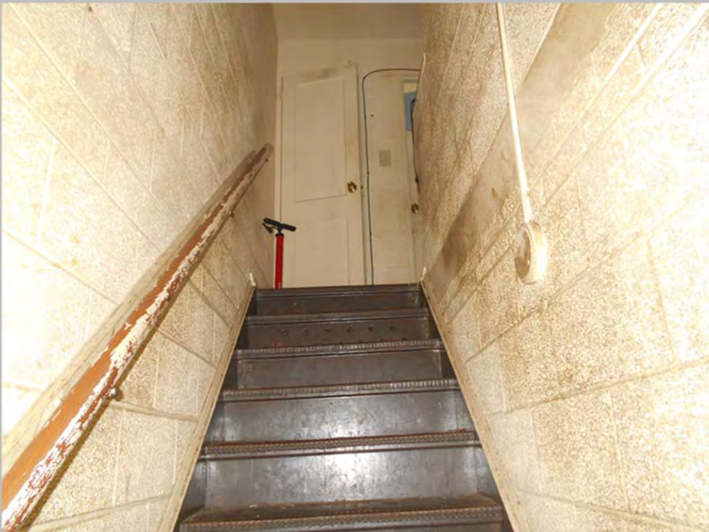
Typical dwelling unit interior stairwell
