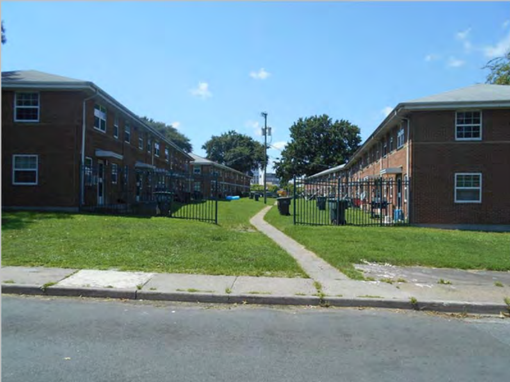
Typical apartment building courtyard
