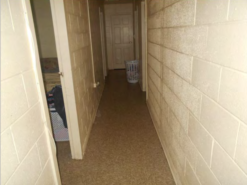
Typical concrete masonry unit interior wall construction
