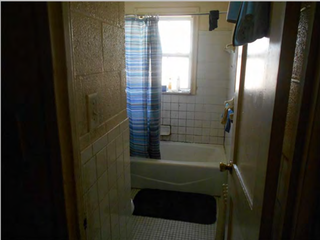
Typical dwelling unit bathroom
