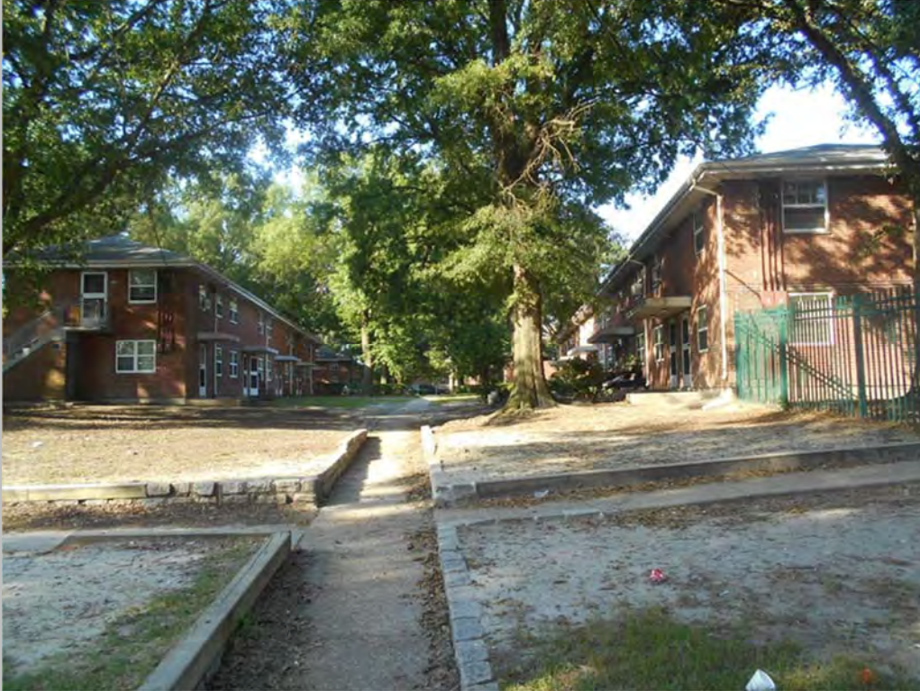
Bare soil and erosion
